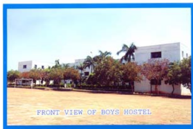
FRONT VIEW OF BOYS HOSTEL
